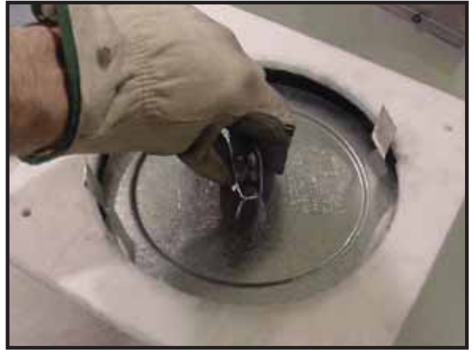
Figure 9.3 Fold the center parts of the retaining band up and use to remove the vent cap.
